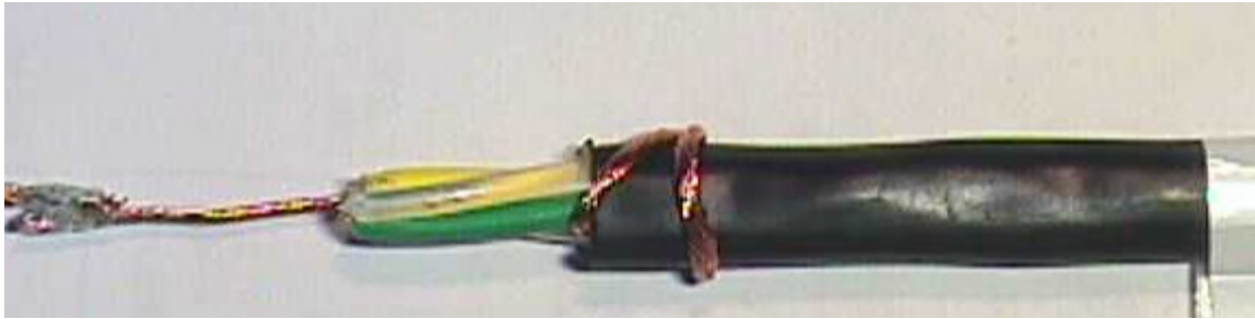
Figure 5 – Bottom view of right side of splice
