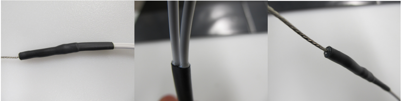
Figure 30 – A completed splice with additional adhesive shrink tube applied.
