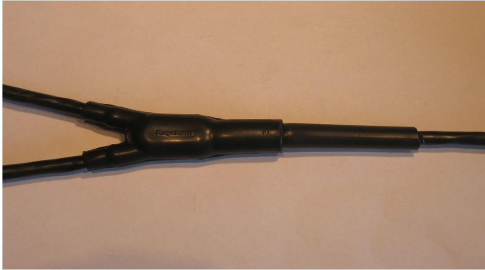
Figure 14 – Finished cable with Raychem Y- Shrink.
