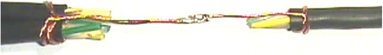
Figure 1 – Drain wire implementation over the entire splice
