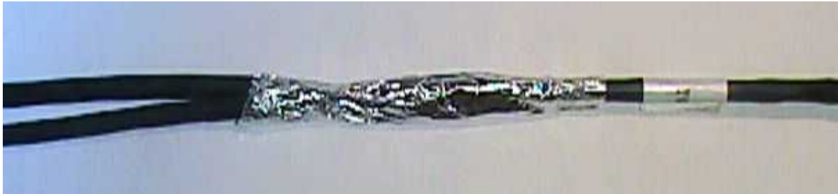
Figure 7 – Cable after being wrapped with foil wrap
