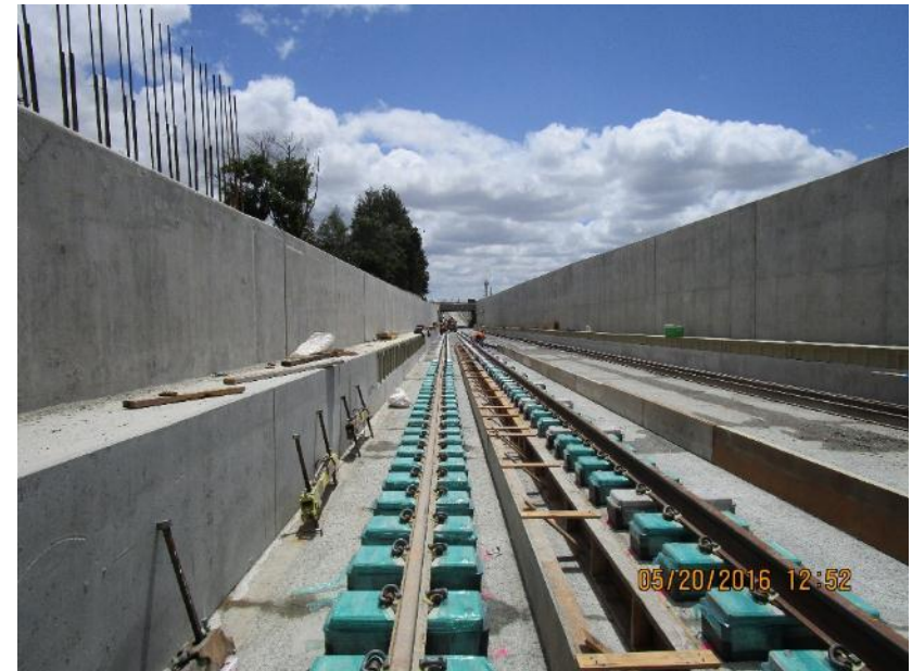
Track installation within the trench at Dixon Landing Road.
