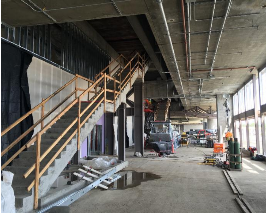
Construction of stairways and interior walls of the Berryessa Station concourse.
