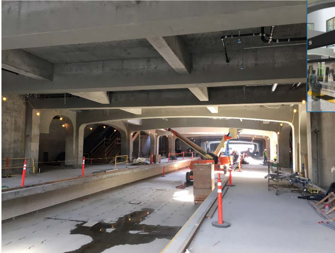
View of the Milpitas Station platform level.
