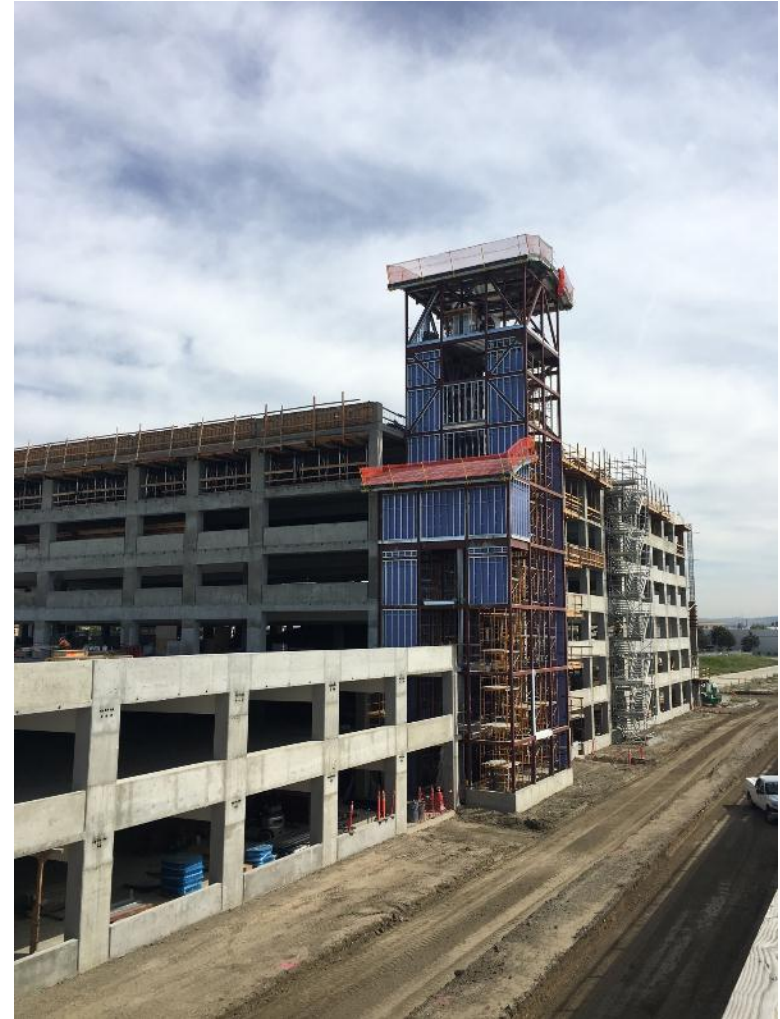
Construction of the Berryessa parking structure elevator tower.
