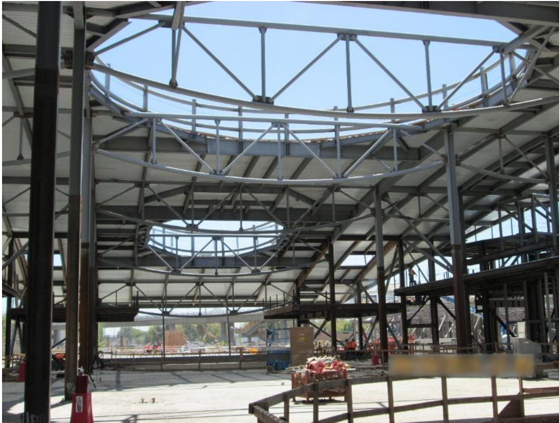
View of the Milpitas Station concourse with steel framing in place.
