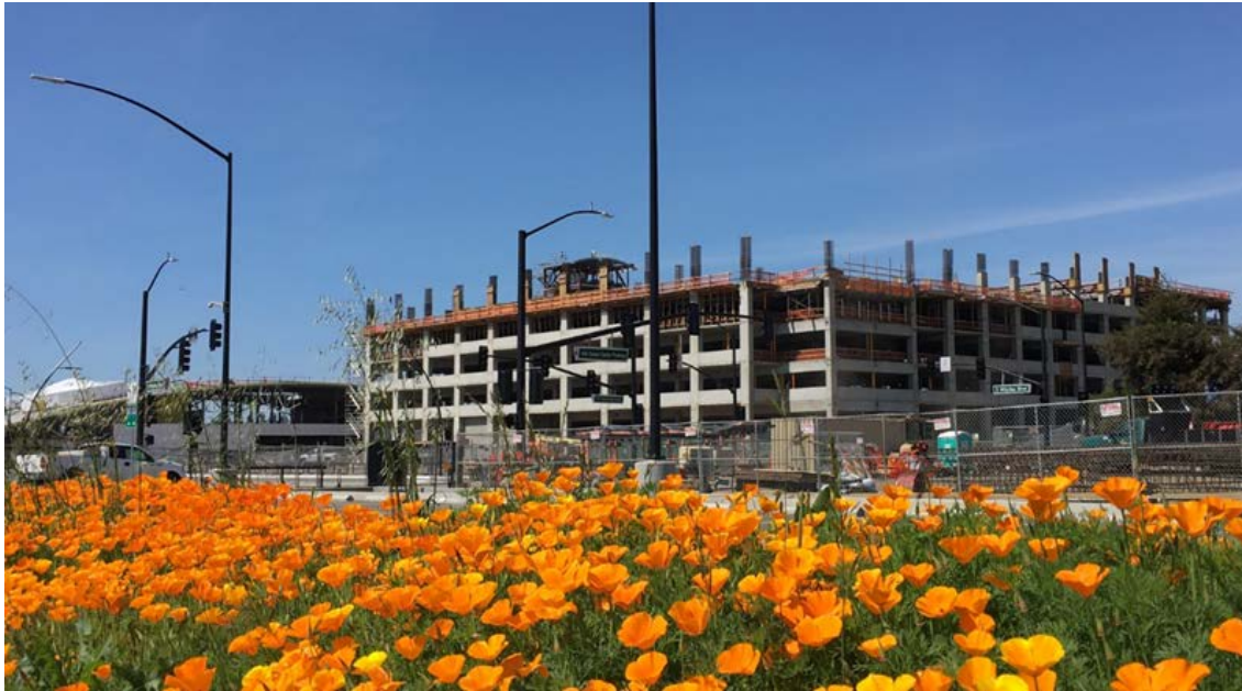
Looking west towards the Milpitas Station and parking structure.
