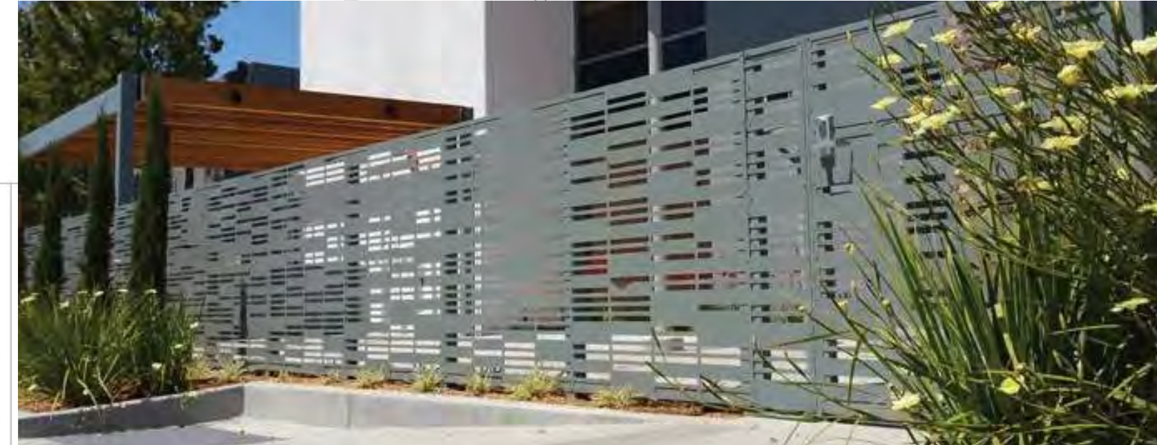
3 PERFORATED STEEL PANEL FENCE/ROLLING GATE (MATCH ARCHITECTURAL SPEC)
